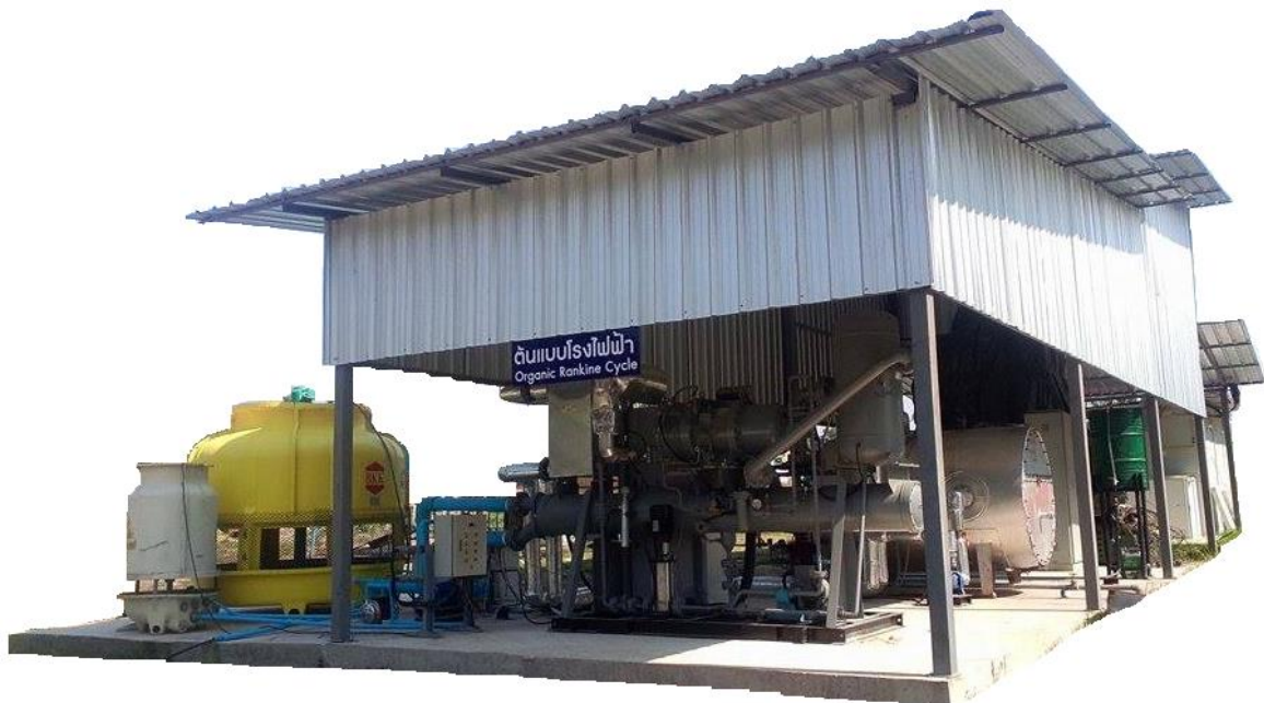
Figure 2 The ORC Prototype with using R-245fa as working fluid
