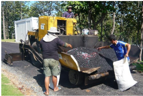
Figure 7 Mixing plastic bag waste with a paving machine
