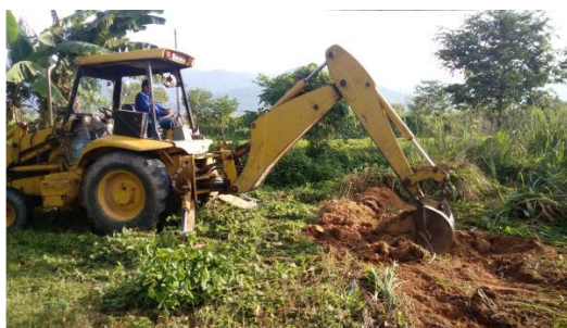
Fig. 6: Pit is dug using JCB excavator.
