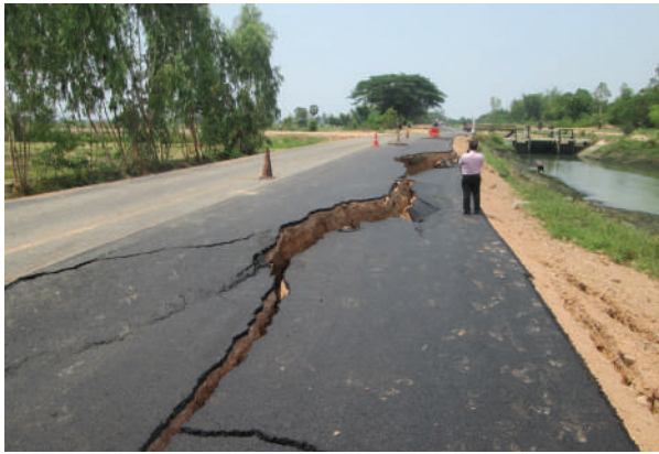
Figure 2: The road collapsed one day after the construction
