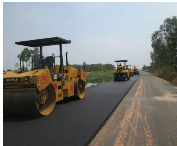
Figure 1: Asphalt concrete surface construction
