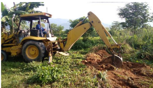
Fig. 6: Pit is dug using JCB excavator.
