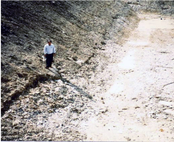
Fig. 36: Lom Sak, Phetchabun Province fish pond, the man stands on the previous bank of the pond where the pond was filled by catastropholess and buried fishes.
