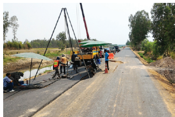
(c) Sampling with standard penetration test (SPT)
