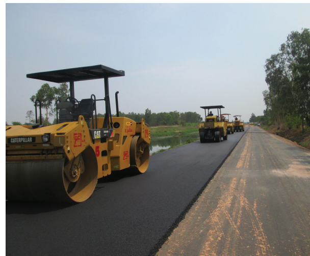
Figure 1: Asphalt concrete surface construction
