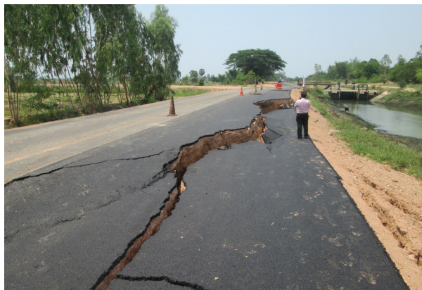
Figure 2: The road collapsed one day after the construction
